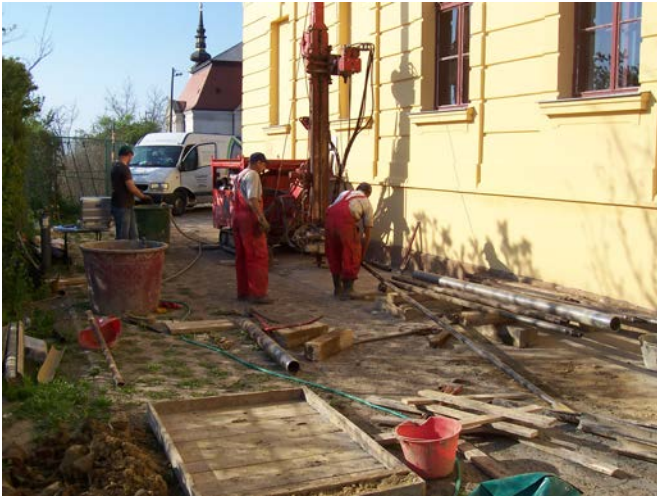
Fig. 3. Preparation of DMT test near high school building.
